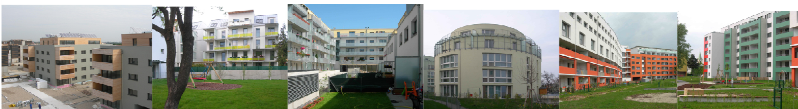
From left to right: Am Muehlweg, Utendorfgasse, Roschegasse, Dreherstrasse, Kammelweg B and E.
