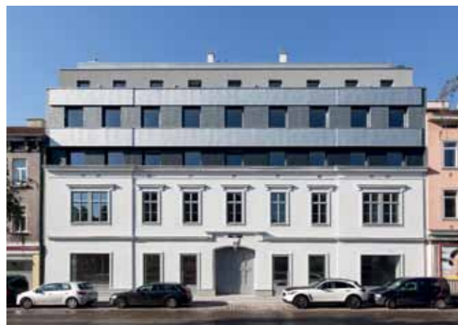
Top floor extensions, where suitable and possible, create new living space.
