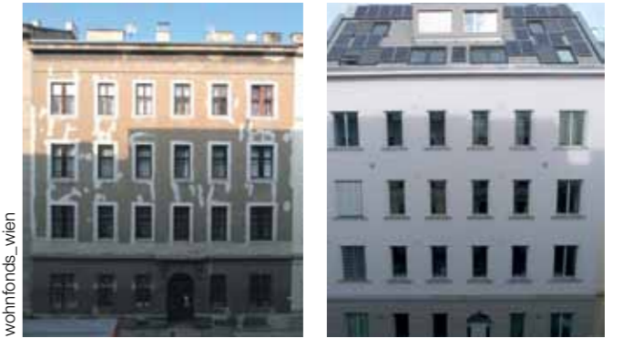
Before and after the innovative refurbishment: The Gründerzeit house at Eberlgasse 3
