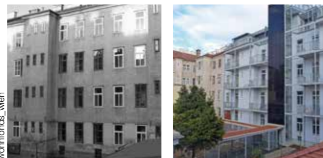
Example: Dopplergasse 5 in the 11th district before and after renovation
