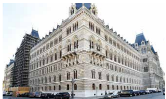
Renovation of the City Hall central risalit
