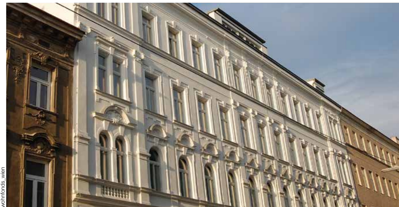
The renovated street façade of the flagship project on Dopplergasse
